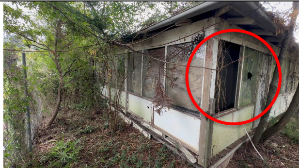
View of the southern façade of the eastern cottage illustrating the overgrown shrubs plantings and trees limiting access and compromising the integrity of footings due to tree root growth. Damaged glazing and missing screens pose a security risk for this unoccupied building
