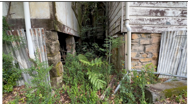
View of the western recess between the western cottage and the link illustrating the damage to the perimeter of the cottages resulting from uncontrolled discharge of rainwater from the roof and gutters. The high moisture levels around the perimeter of the cottages has resulted in some settlement of perimeter walls and piers.
