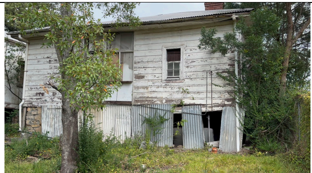
View of the western end of the northern façade illustrating the lack of weather protecting and security with open windows and poorly secured later sheeting.
