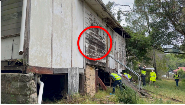
View of the northern facades illustrating the lack of protection of the wall cladding materials.
