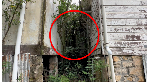
View of the western recess between the western cottage and the link illustrating the damage to the original weatherboarded bay window resulting from ongoing discharge of rainwater onto this section of the façade from the roof. Invasive plant growth due to high moisture conditions limited access.
