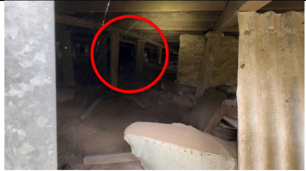
View of the subfloor area from the north-western corner illustrating the condition of the timber piers, bearers and joists.
