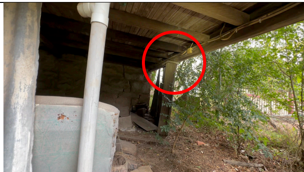
View of the subfloor area from the north-western corner illustrating the hardwood timber piers with galvanised iron ant caps that will have provided some protection from termite attack.
