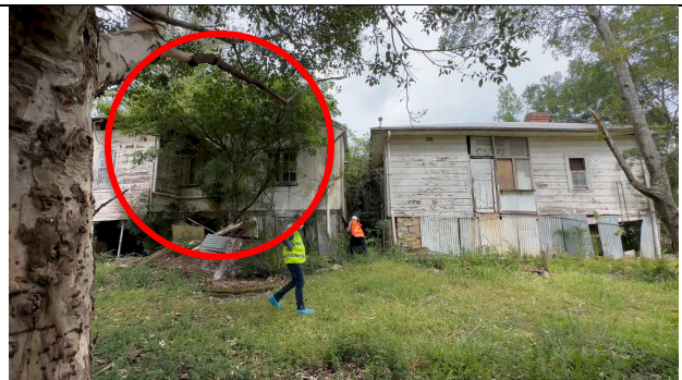
View looking south towards the NW end of the cottages illustrating the proximity of some trees and vegetation posing a physical risk and likely to raise moisture levels in and around the building with damaging consequences to the fabric.
