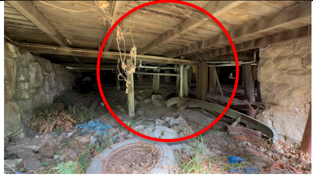
View of subfloor area from the north-eastern corner illustrating that the apparent damage is focused on the perimeter of the cottages resulting from uncontrolled discharge of stormwater around the perimeter of the building.
