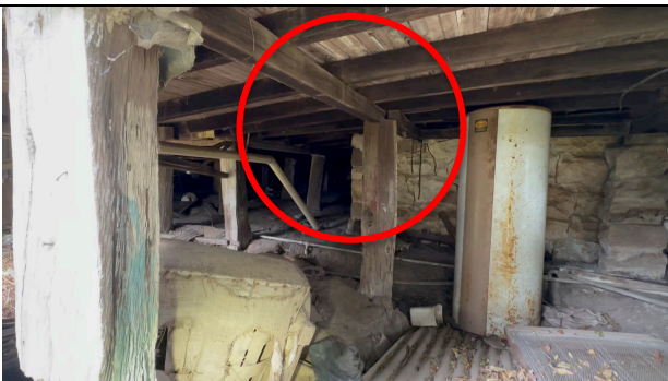
View of the subfloor area from the north-western corner illustrating the condition of the stone footings for fireplaces and the hardwood piers located away from the perimeter of the building appear to be in fair condition.
